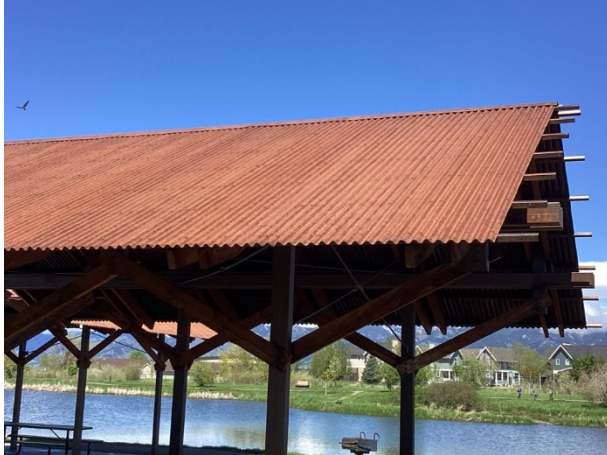
Corrugated steel roofing at pavilion
