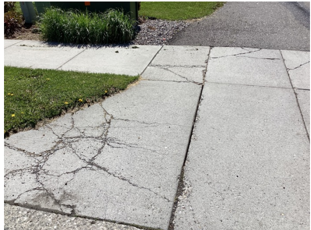
Cracks and spalls at apron
