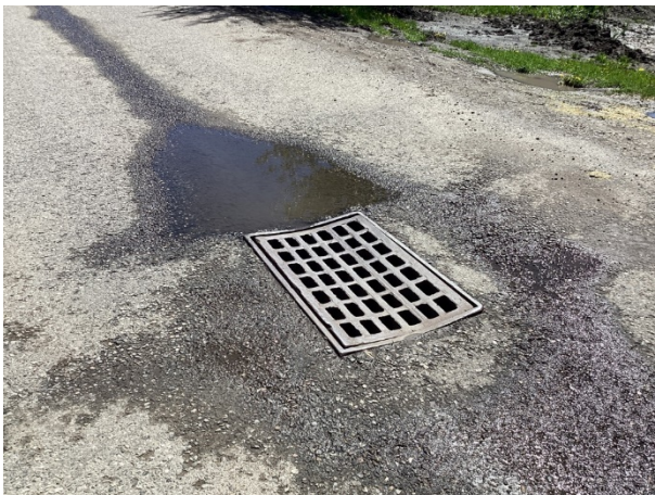
Poor drainage due to pavement settlement near catch basin
