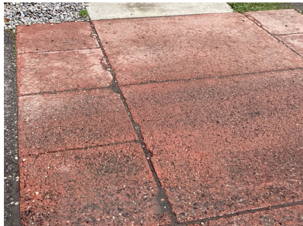
Sidewalk spalls
