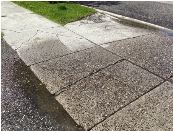
Cracks and spalls at apron
