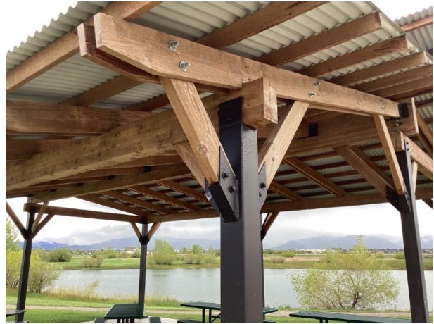
Steel and wood framing
