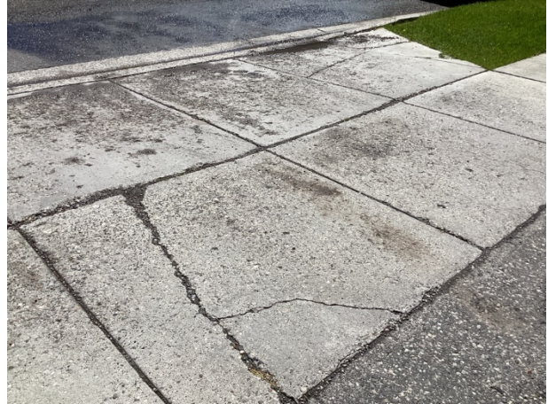
Cracks and spalls at apron
