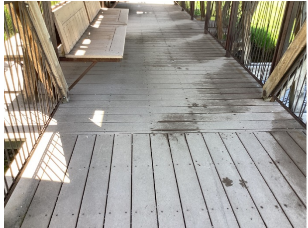
Composite decking at bridge
