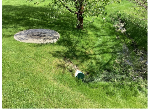
Storm water pipe at retention basin
