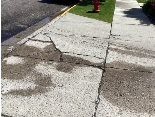
Large settlement cracks at apron
