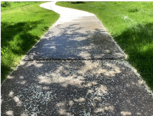
Sidewalk trip hazard
