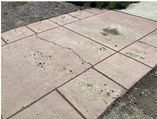
Sidewalk cracks
