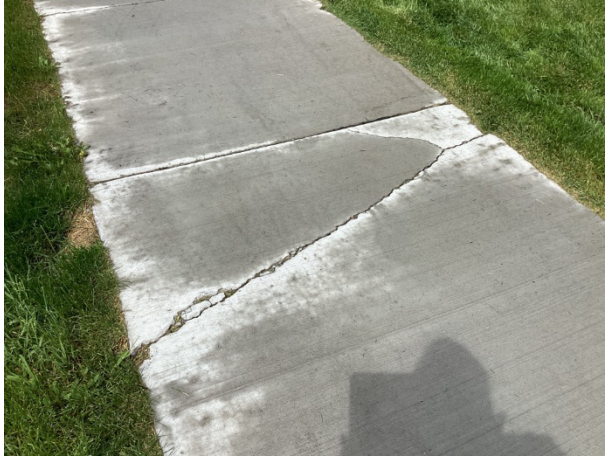
Cracks and spalls at sidewalk at Leiden Lane
