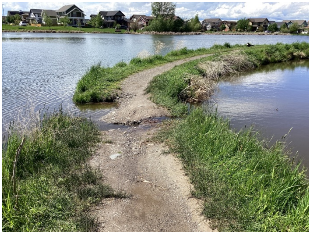
Shoreline erosion at east embankment
