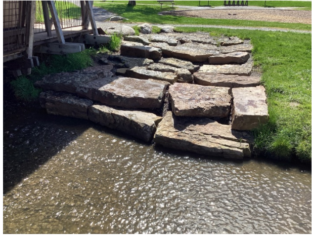
Previous shoreline stabilization repair
