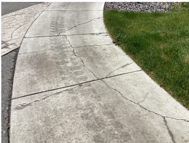
Sidewalk cracks at Arnhem Way
