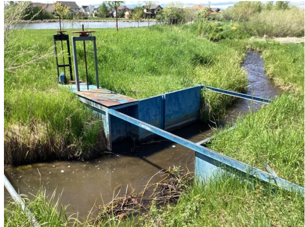
Sluice gate control structure
