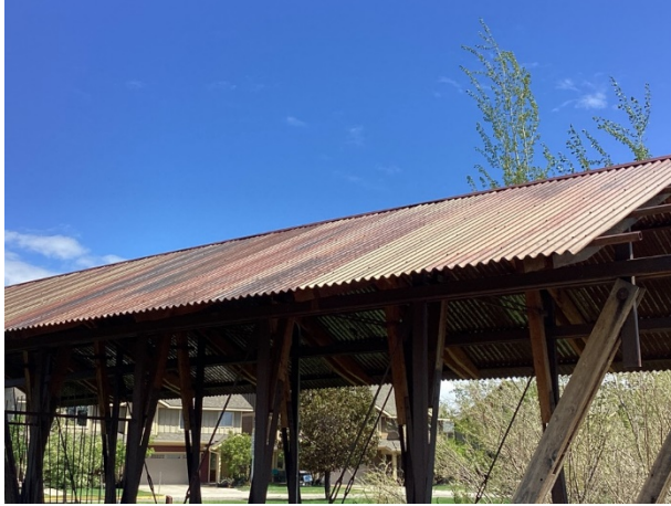
Corrugated steel roof
