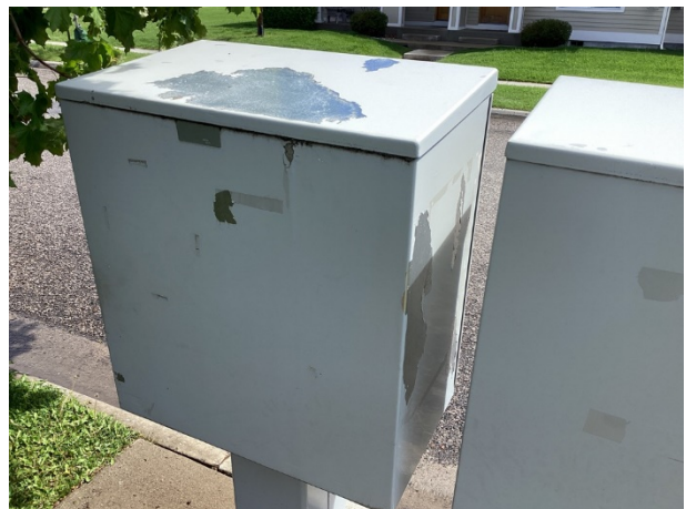
Mailbox station finish deterioration
