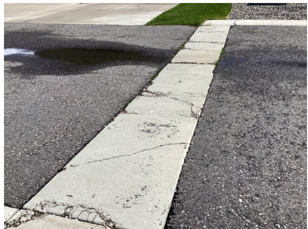
Curb cracks and spalls at Deft Way
