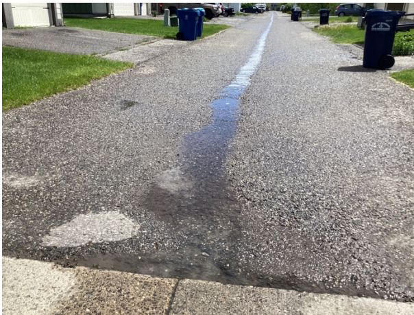
Pavement deterioration near apron
