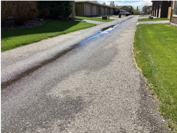
Centerline drainage at alley
