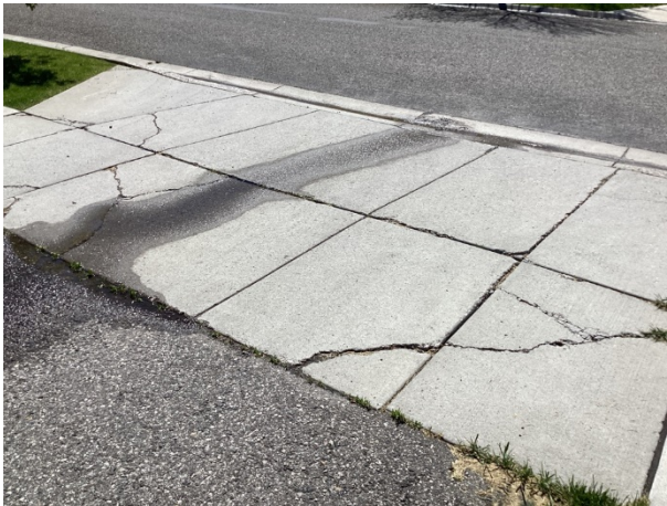
Cracks at apron
