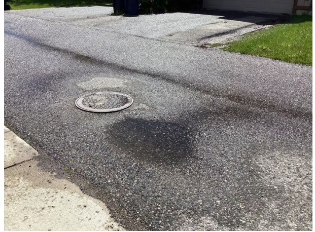
Pavement settlement near manhole cover
