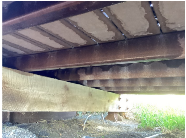
Bridge steel support and wood support joist
