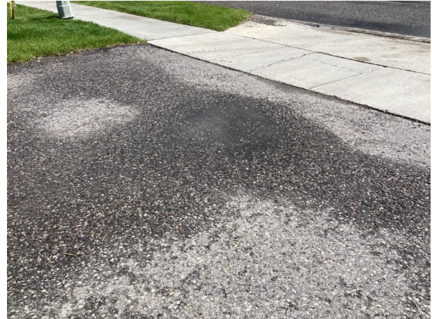
Pavement settlement and ravels
