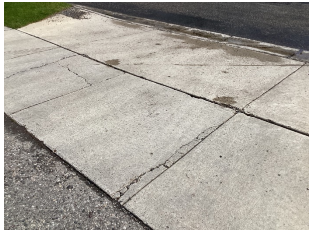
Cracks at apron
