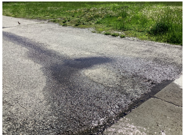
Pavement settlement and deterioration near apron
