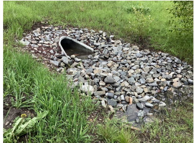
Storm water culvert and rip rap
